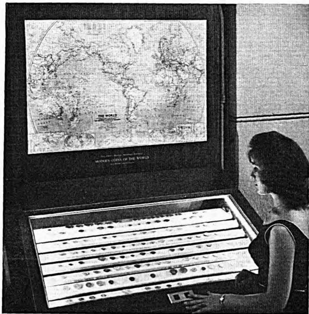
Fig. 16.—This semiautomatic case is used for the display of about 800 coins. It has 40 trays suspended between continuous chain devices. By pushing an electrical contact visitors may move into the field of view any tray they wish to examine
